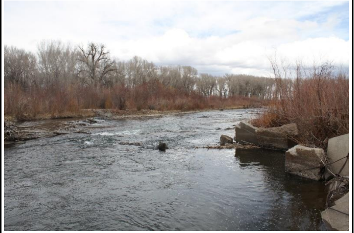
Headgate and diversion dam
