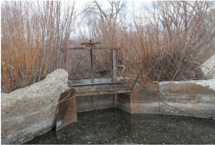
Headgate looking downstream
