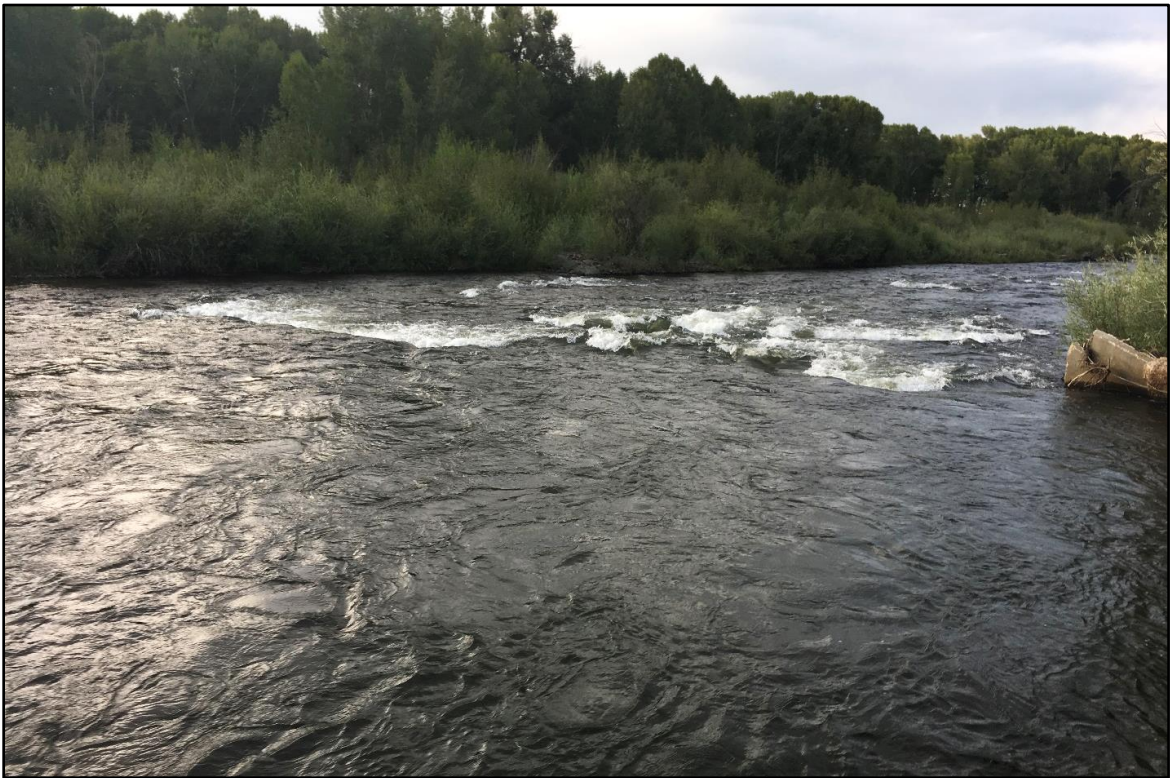
Diversion dam looking downstream post-2019 runoff
