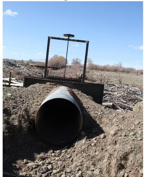
Headgate and trash rack structure
