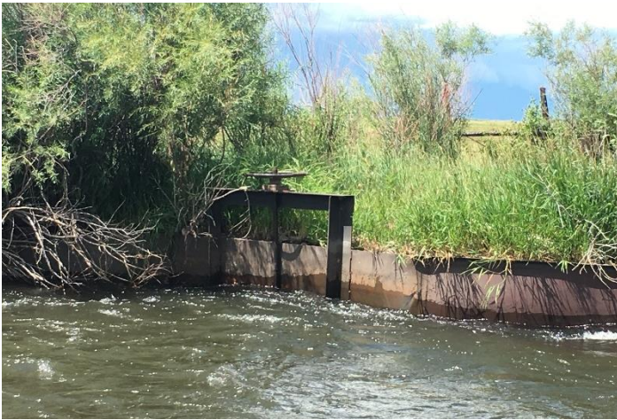
Headgate looking downstream
