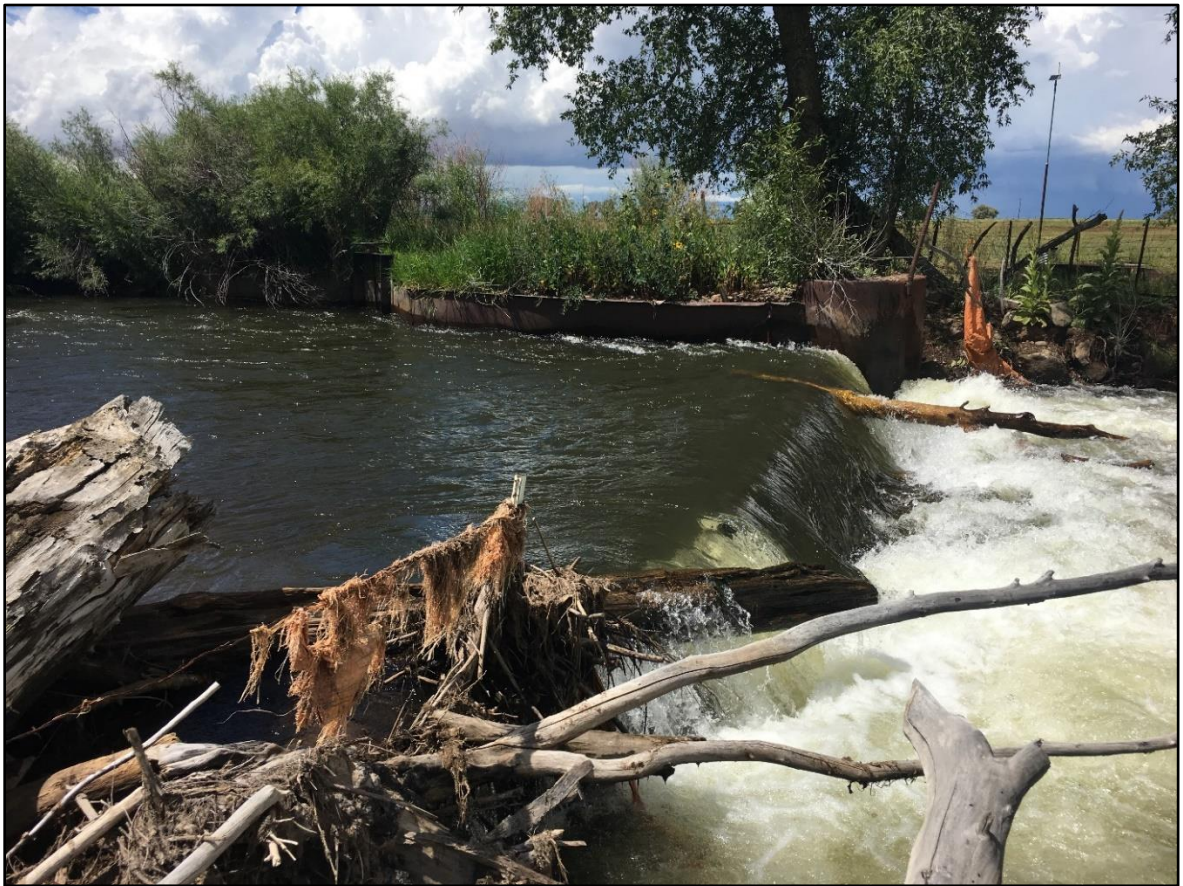
Diversion dam and headgate (post-2019 runoff)
