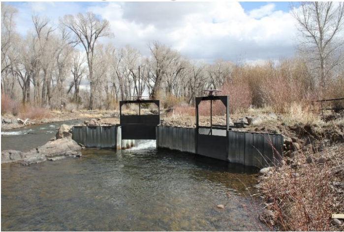
Headgate looking downstream
