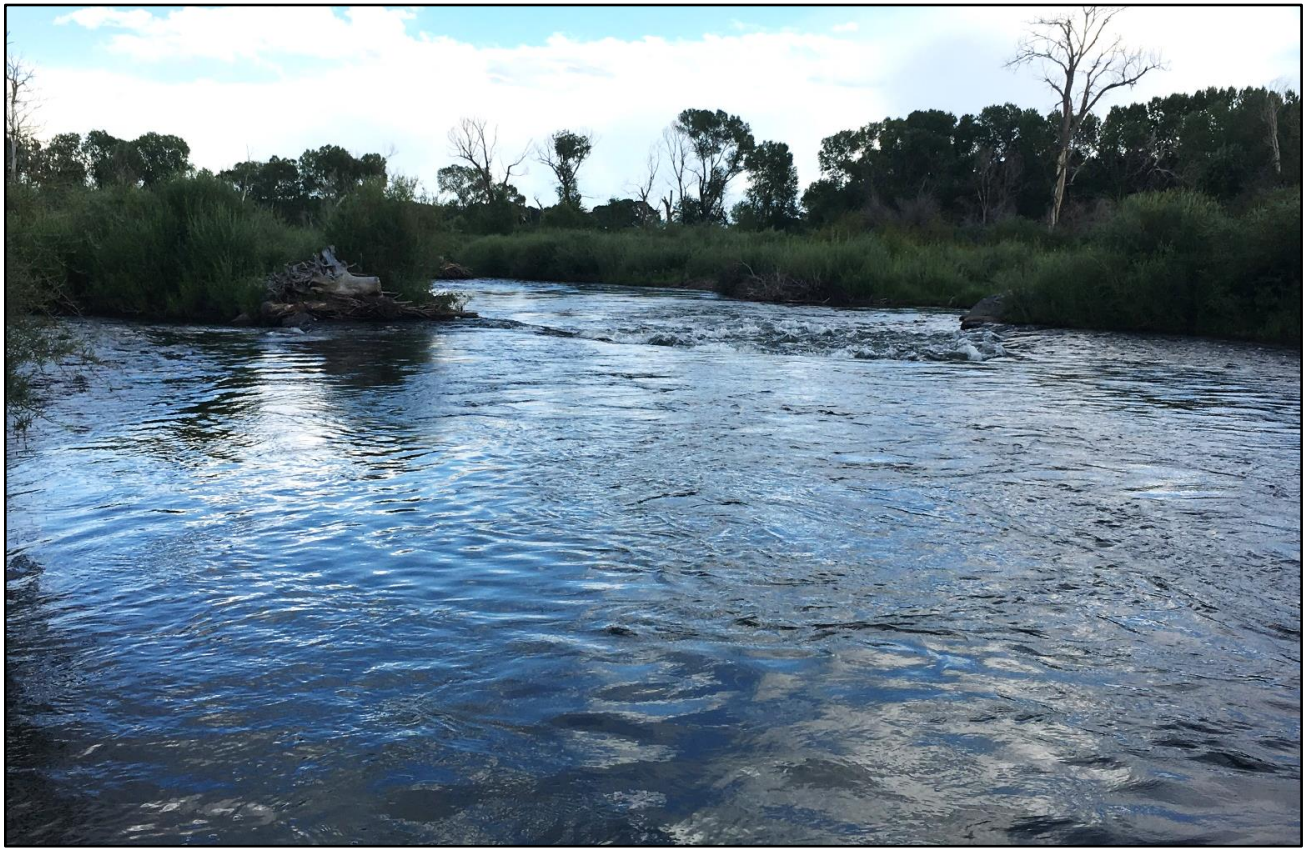
Diversion dam on Conejos River looking downstream
