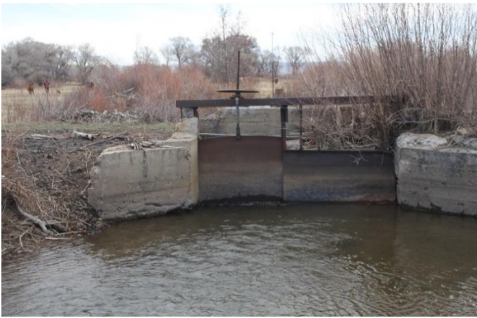
Headgate looking downstream
