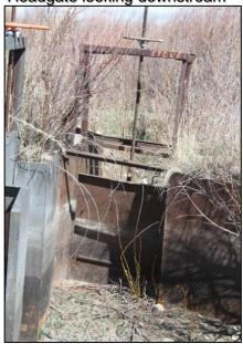
Headgate and sluice gate
