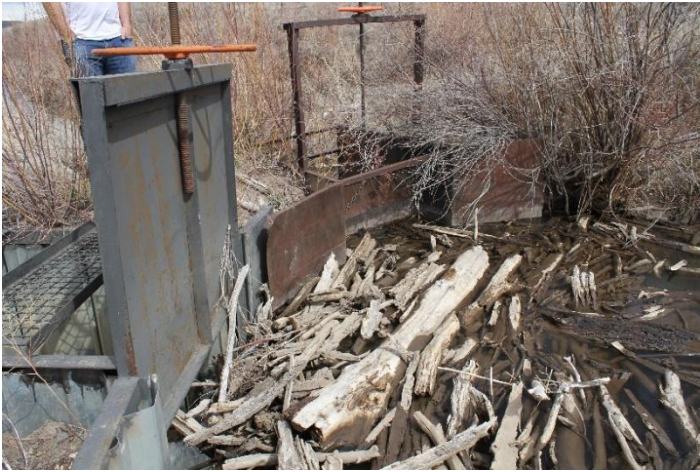
Headgate looking downstream
