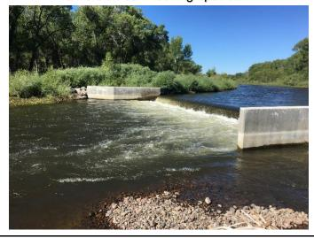
Diversion dam and sluice gate
