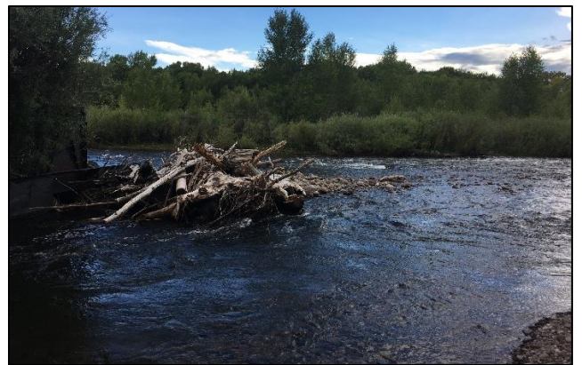
Diversion dam on Conejos River (post-runoff)
