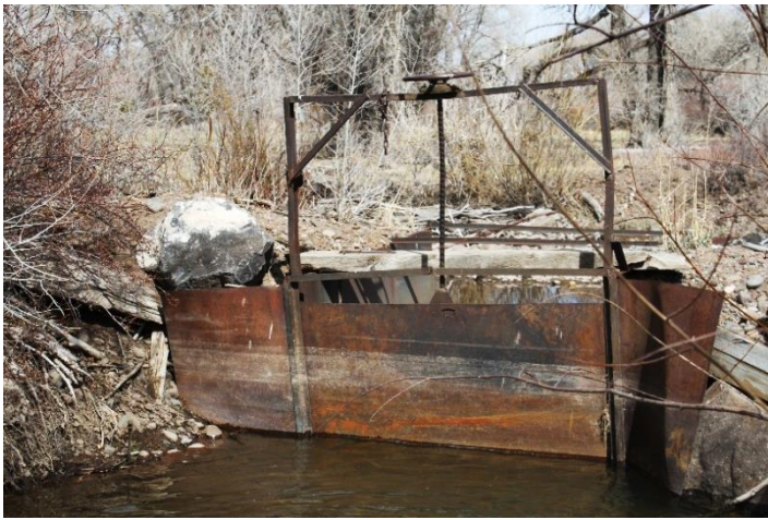
Headgate looking downstream (pre-runoff)
