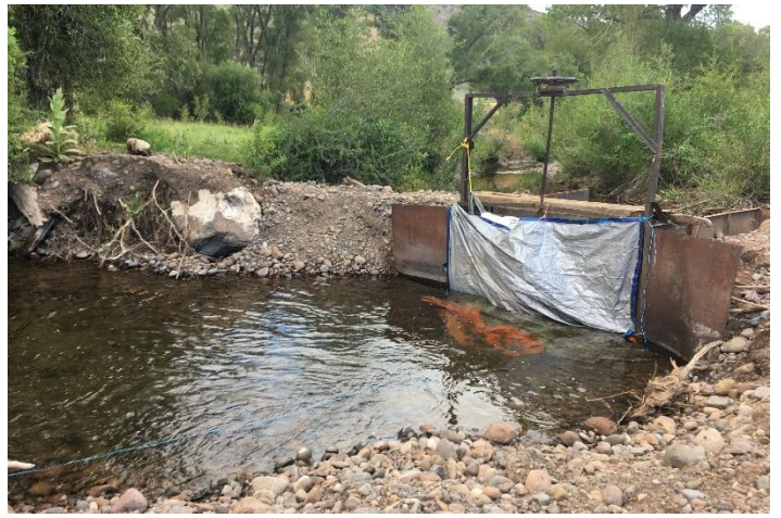
Headgate looking downstream (post-runoff)
