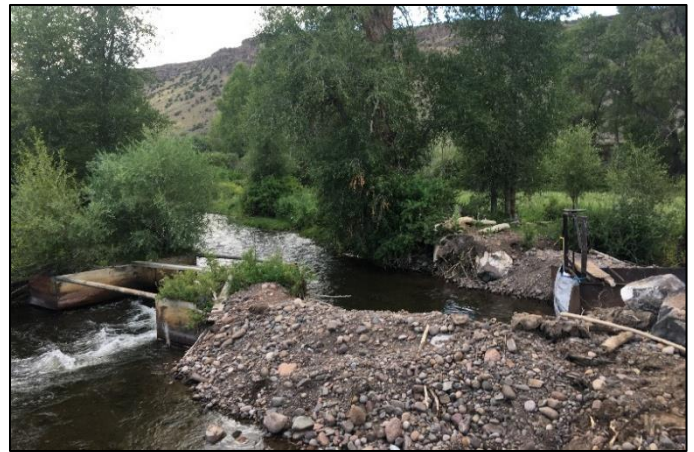
Headgate and overflow structure post-runoff 2019 (looking upstream)
