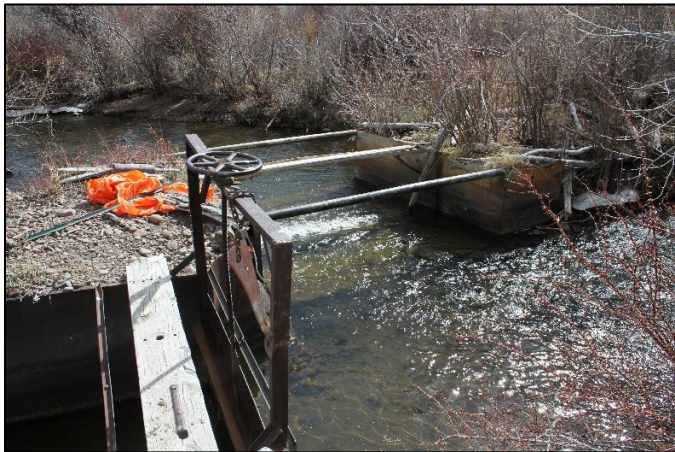
Headgate and overflow structure pre-runoff 2019 (looking downstream)
