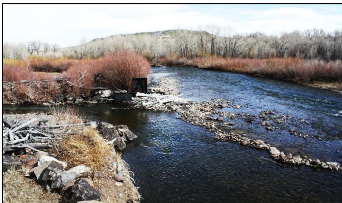
Diversion dam on Conejos River (pre-runoff)
