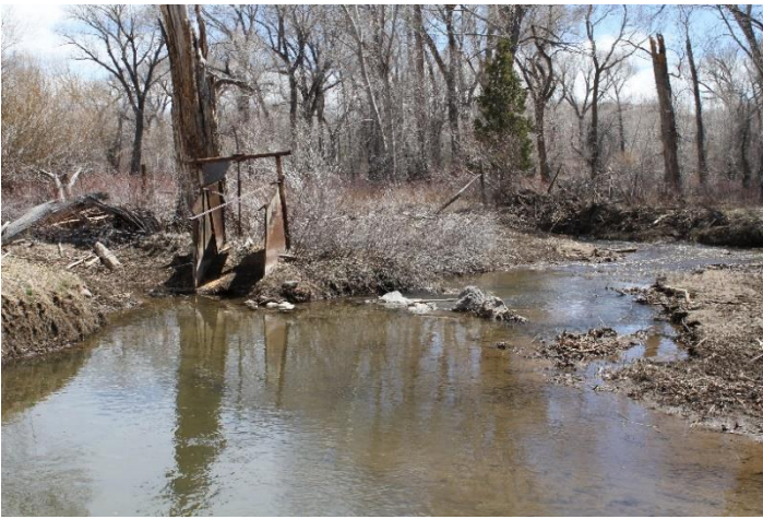
Headgate and diversion dam
