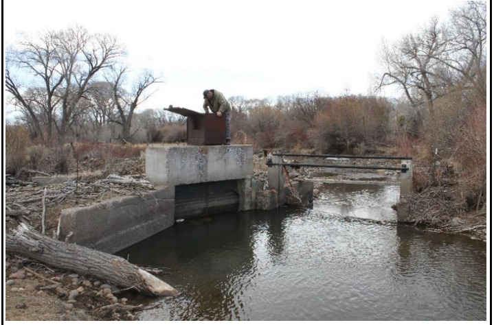
Headgate and diversion dam
