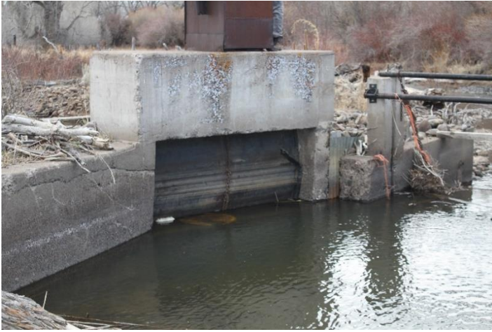
Headgate looking downstream
