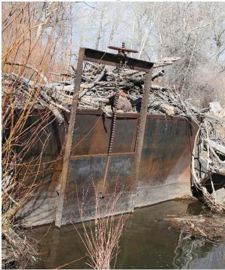
Headgate looking downstream
