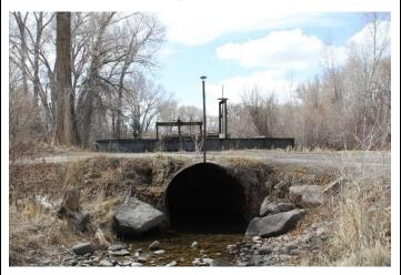
Feeder channel upstream of headgate
