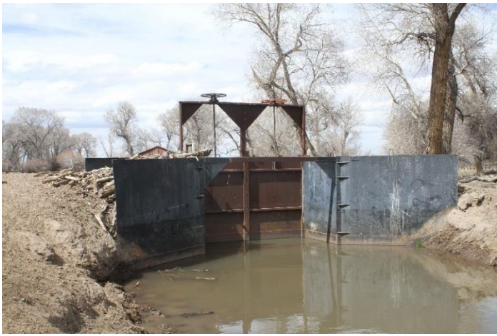
Headgate looking downstream
