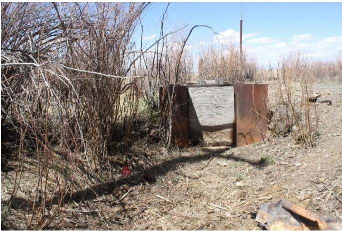
Headgate looking downstream
