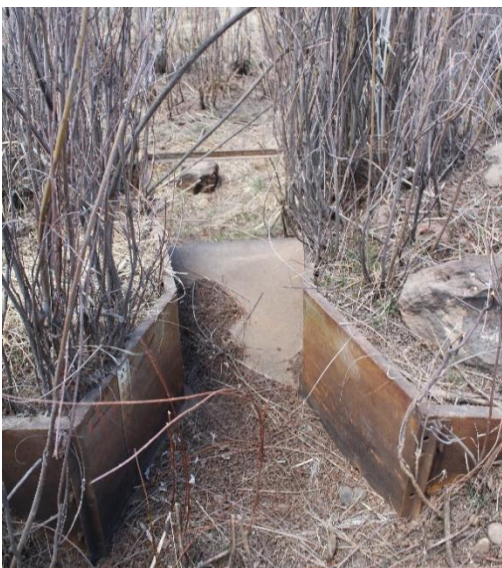
Parshall flume looking downstream
