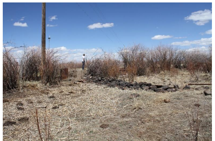
Headgate and diversion dam
