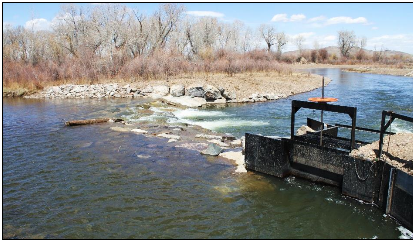
Figure 2.1: Del Puerticito Ditch diversion on the Conejos River.
