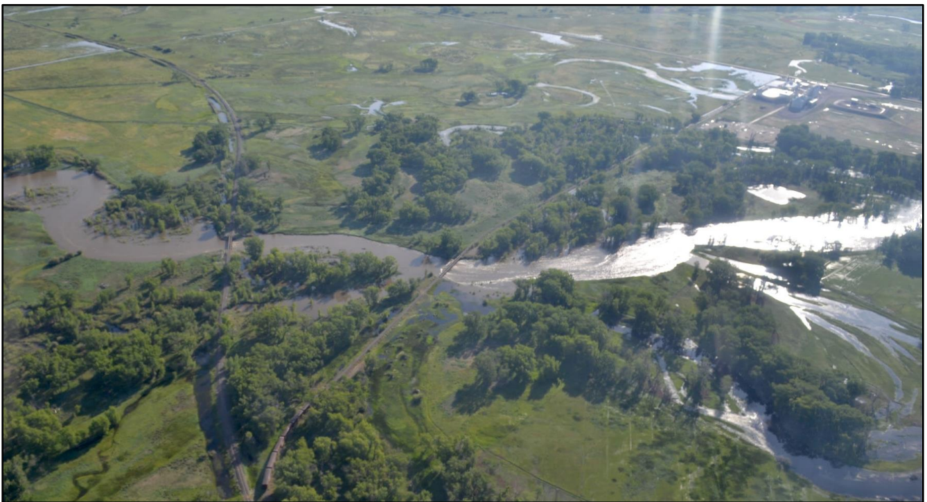
Figure 2.13: Railroad lines and bridges crossing the Rio Grande near flood stage, June 2019.
