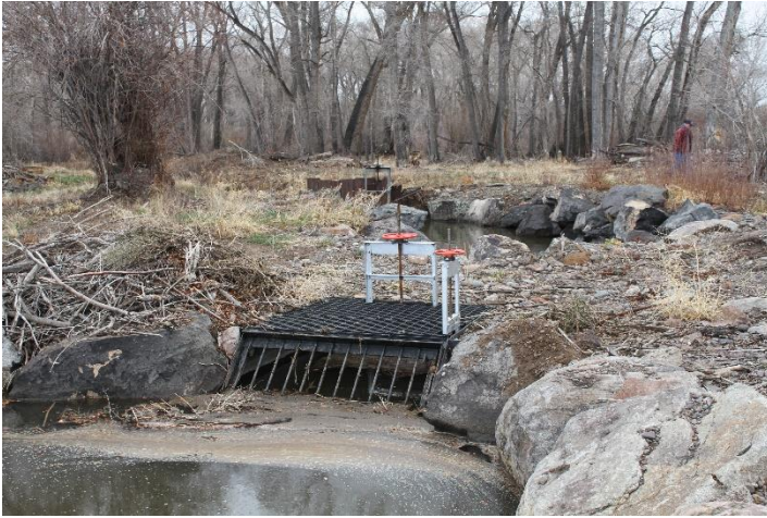
Headgate looking downstream
