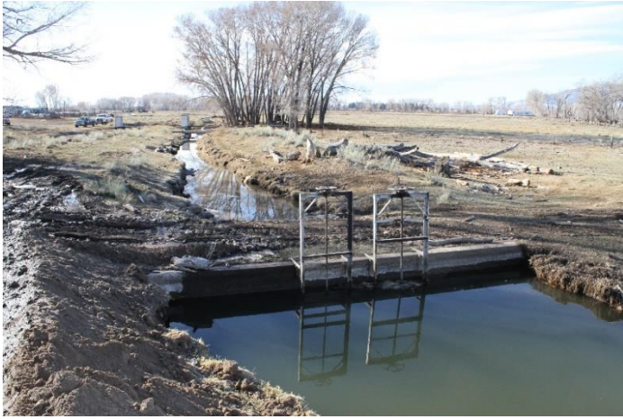
Headgate looking downstream
