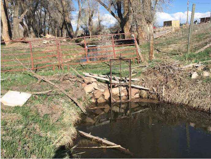
Headgate looking downstream
