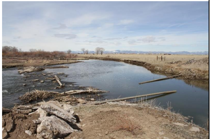
Diversion dam looking upstream
