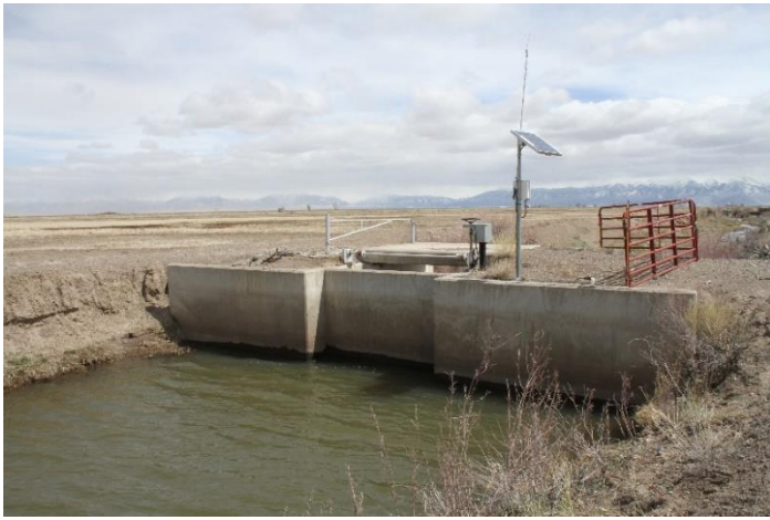
Headgate looking downstream
