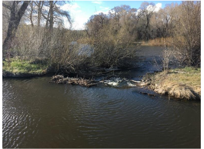
Overflow channel just upstream of headgate
