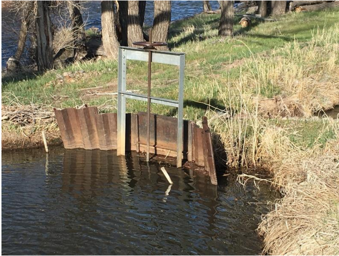
Headgate looking downstream
