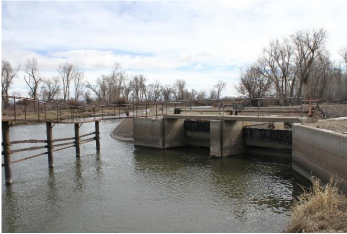
Headgate on the Rio Grande
