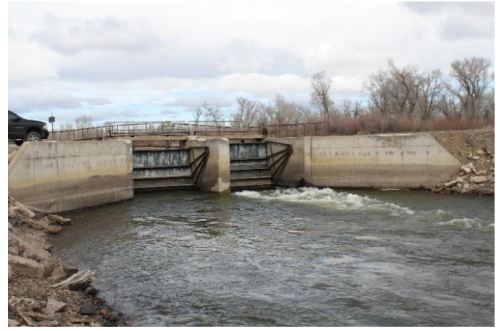
Headgate outlet (on Rio Grande)
