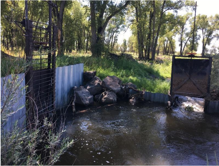
River headgate looking downstream
