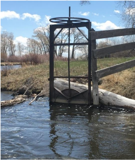
Headgate looking downstream
