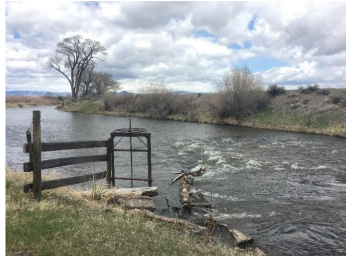
Headgate and diversion dam
