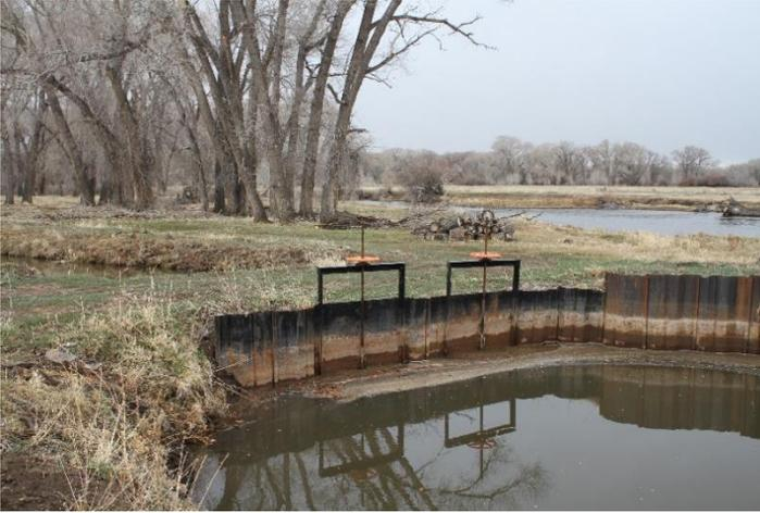
Headgate outlet and adjustment gates
