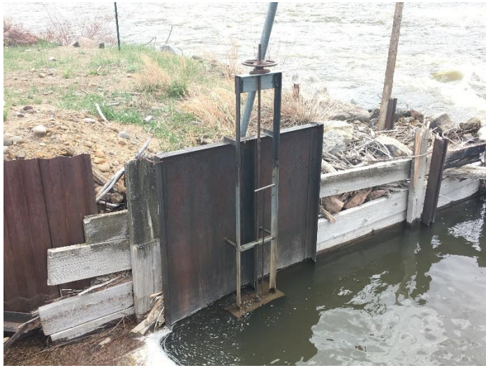
Headgate looking downstream
