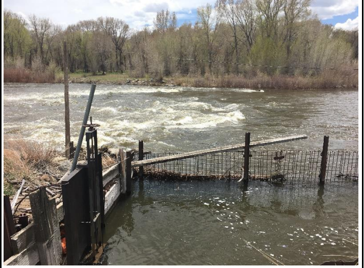
Headgate and diversion dam
