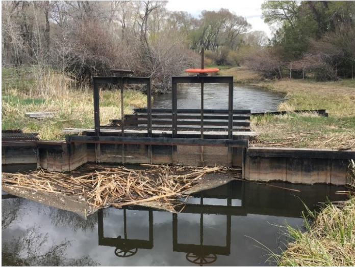
Headgate looking downstream
