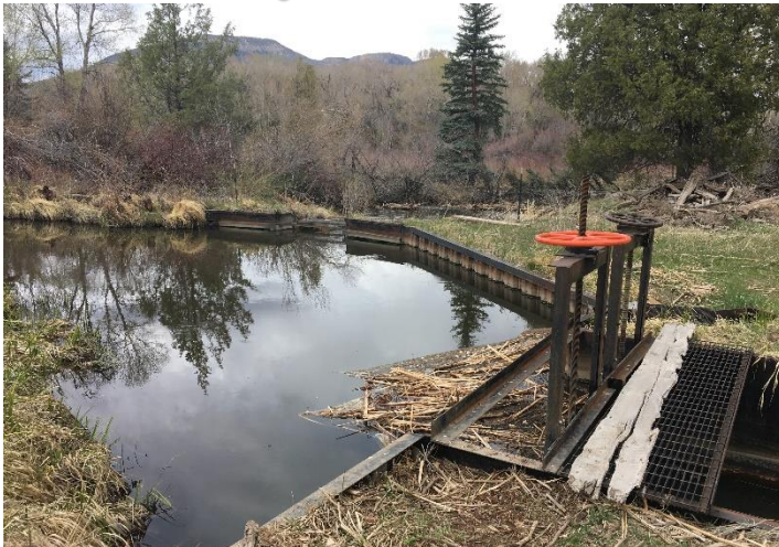
Main headgates and overflow channel
