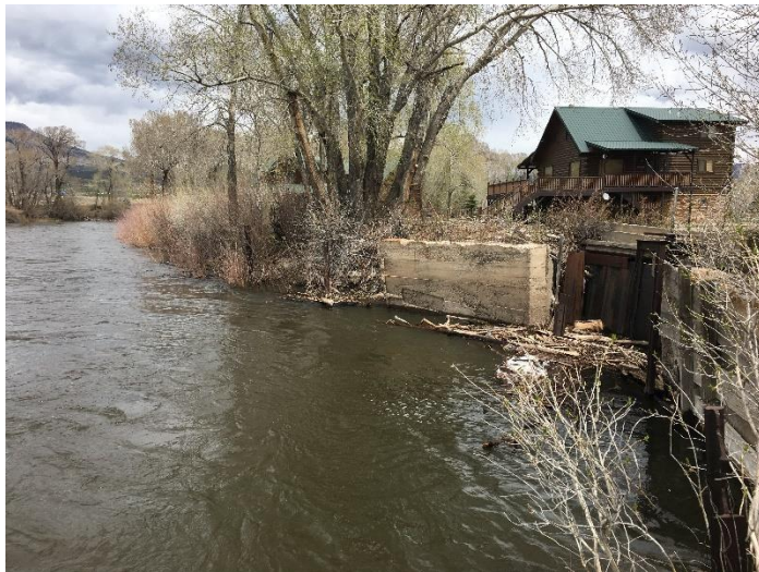
Main headgates and overflow channel
