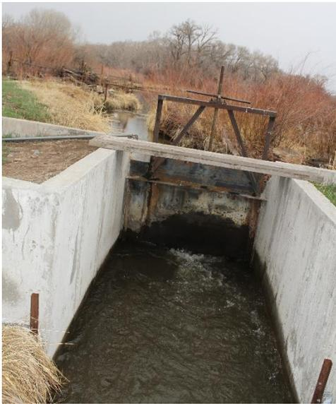
Diversion dam and feeder ditch
