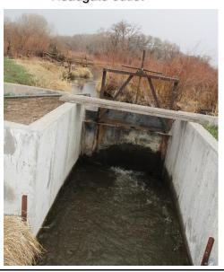
Diversion dam and feeder ditch
