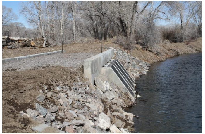
Trash rack looking upstream
