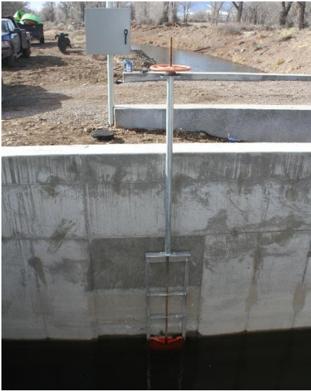
Headgate looking downstream
