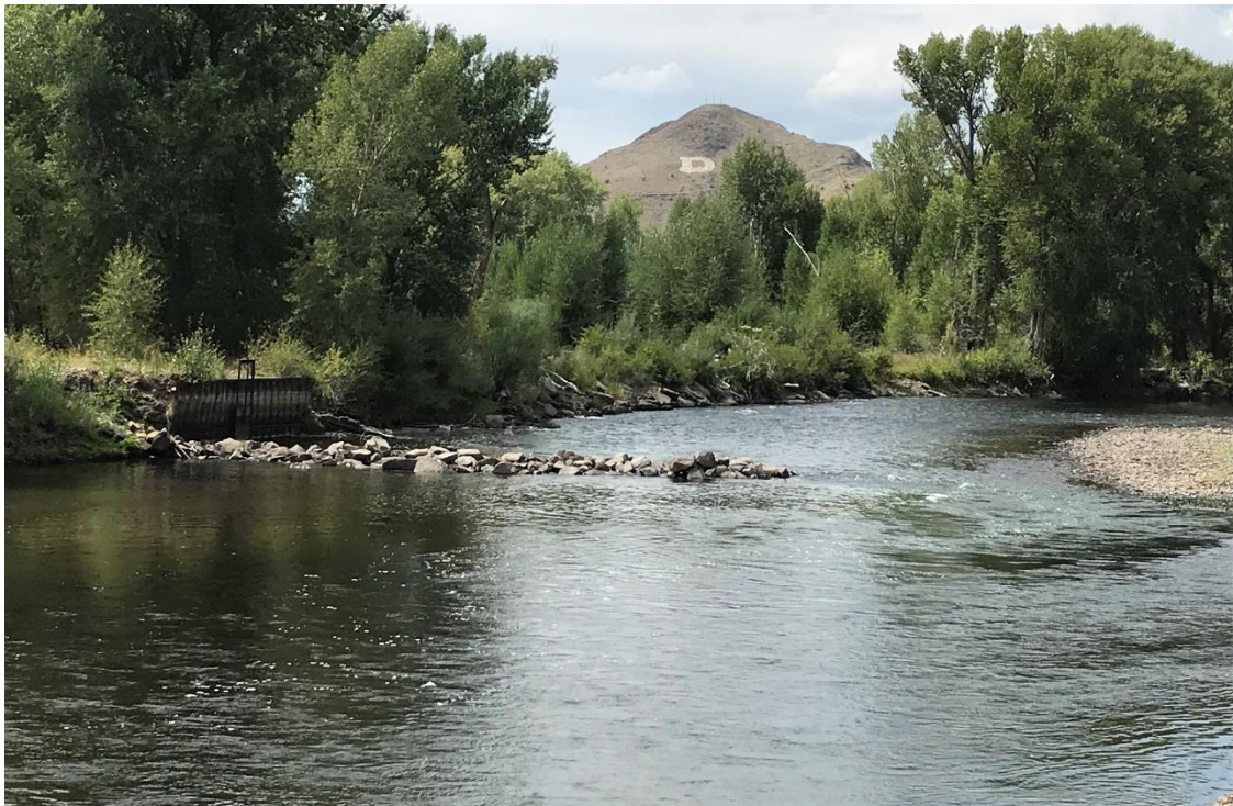
Headgate and diversion dam looking upstream
