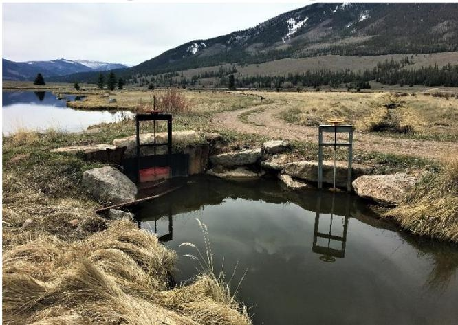
Diversion dam and sluice gate
