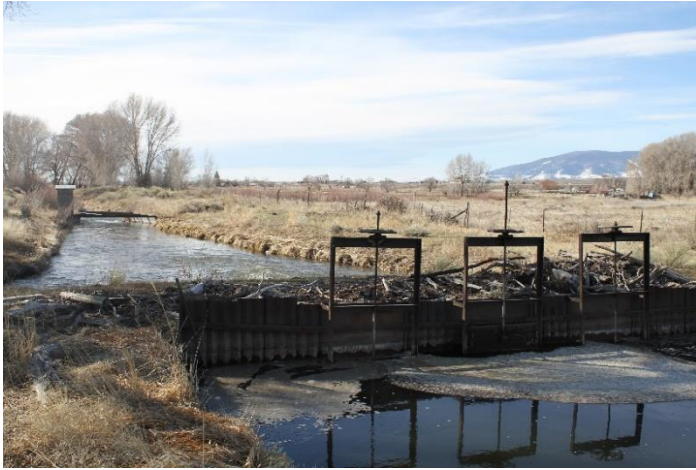
Main headgate looking downstream
