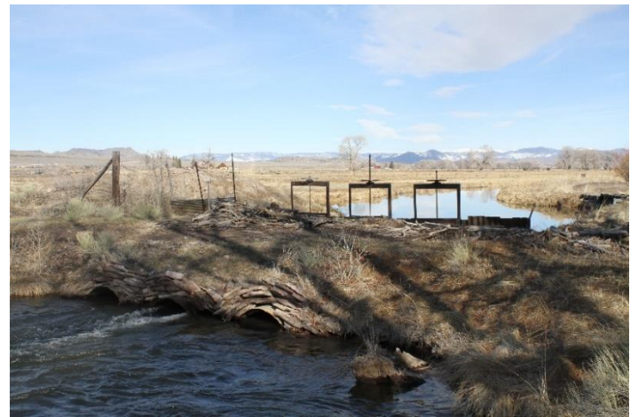
Main headgate outlet
