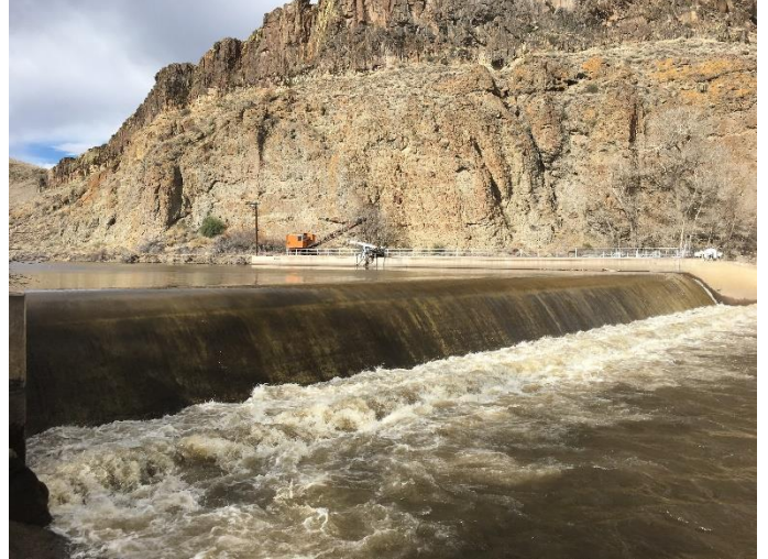
Headgate and diversion dam
