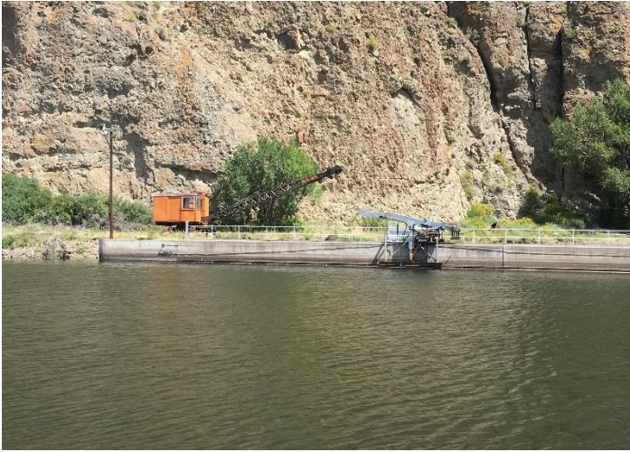
Headgate looking downstream
