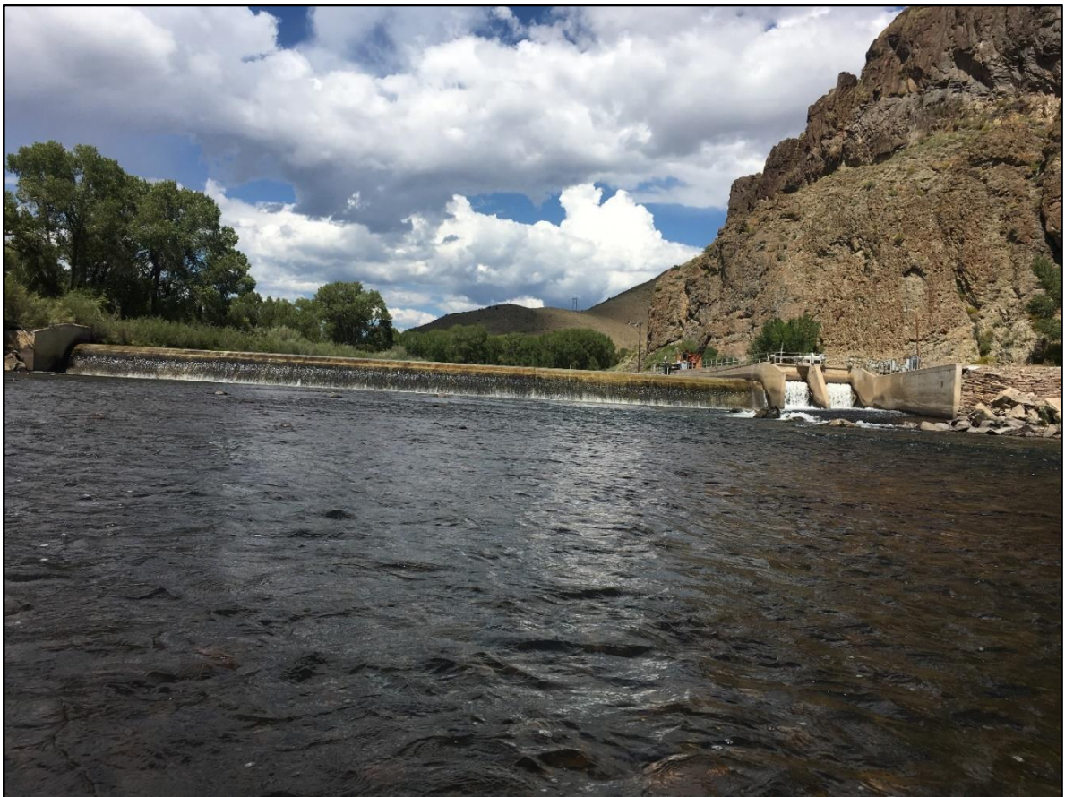
Rio Grande Canal diversion dam looking upstream
