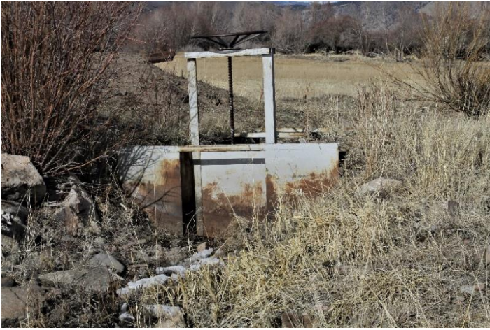
Headgate looking downstream
