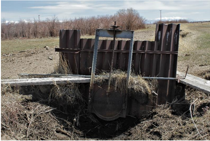
Headgate looking downstream
