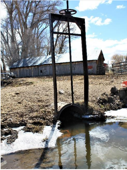
Headgate looking downstream
