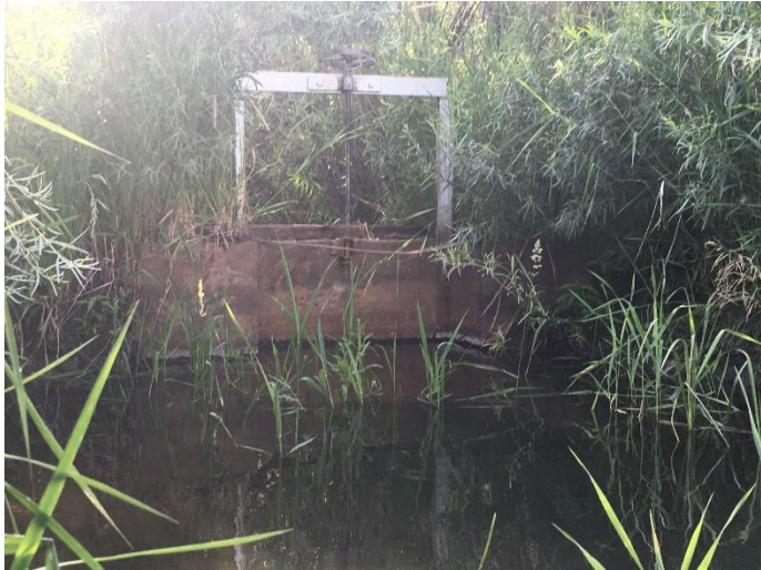
Headgate looking downstream
