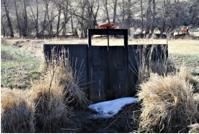
Headgate looking downstream
