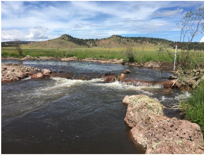
Bank stabilization upstream of headgate
