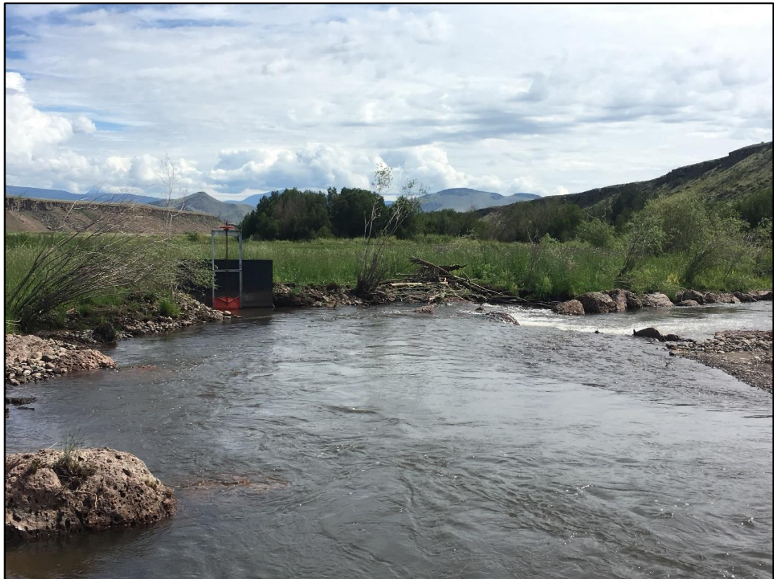
New headgate looking downstream
