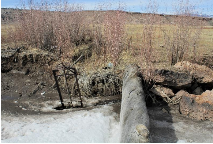
Old headgate looking downstream
