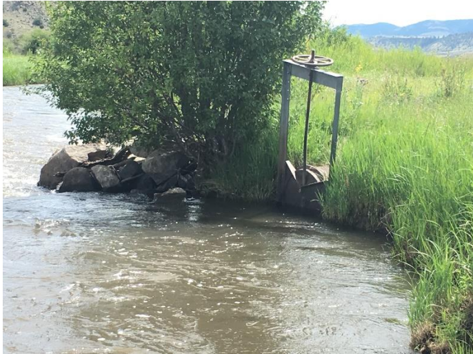
Headgate looking downstream
