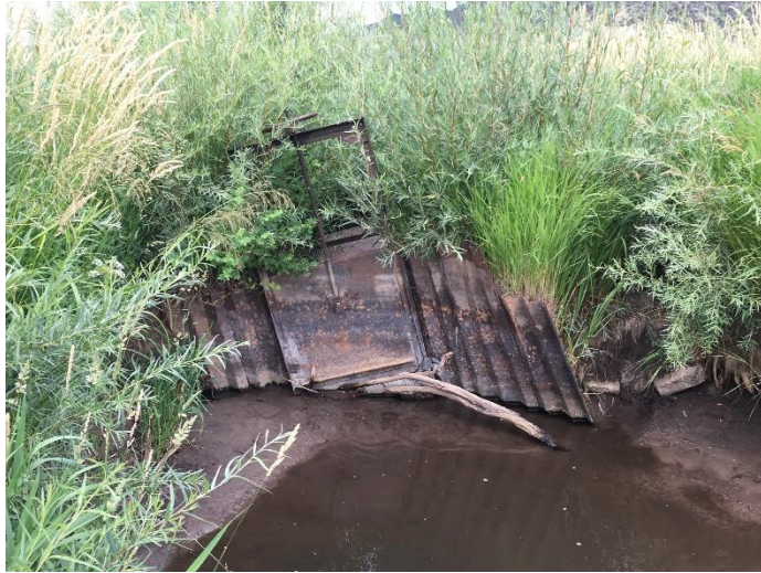
Headgate looking downstream
