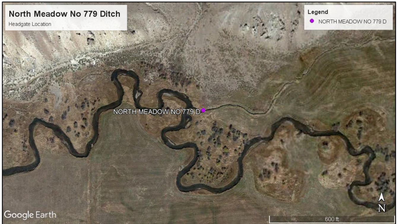
North Meadow No 779 Ditch headgate location
