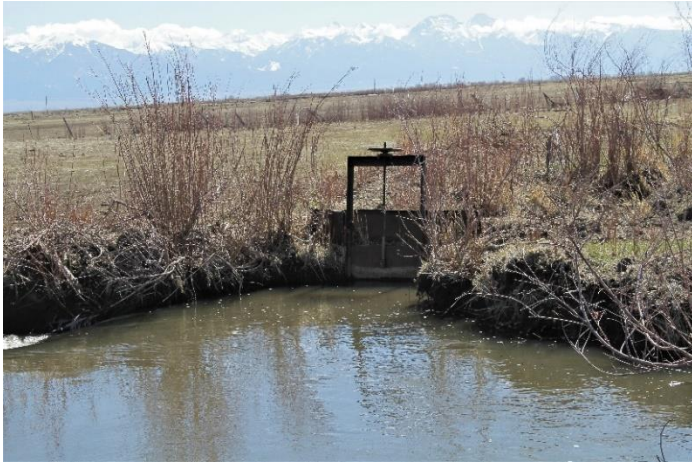
Headgate looking downstream
