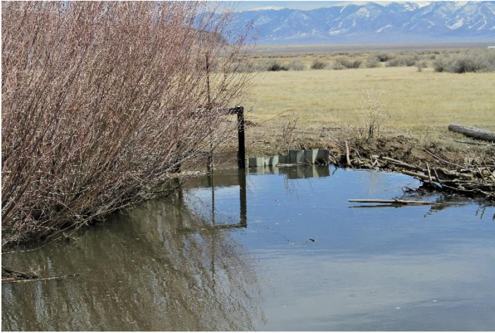
Headgate looking downstream
