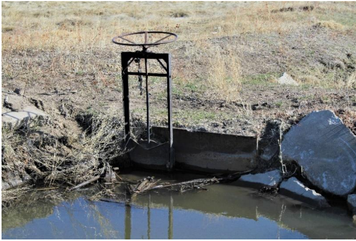
Headgate looking downstream
