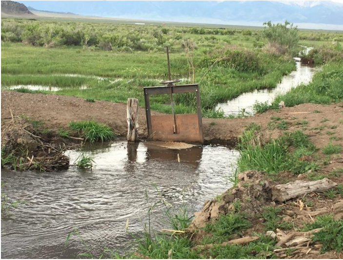
Headgate looking downstream
