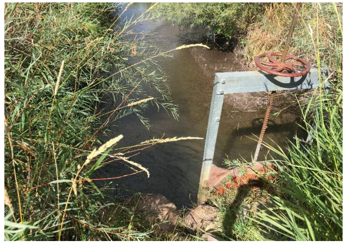
Headgate looking upstream
