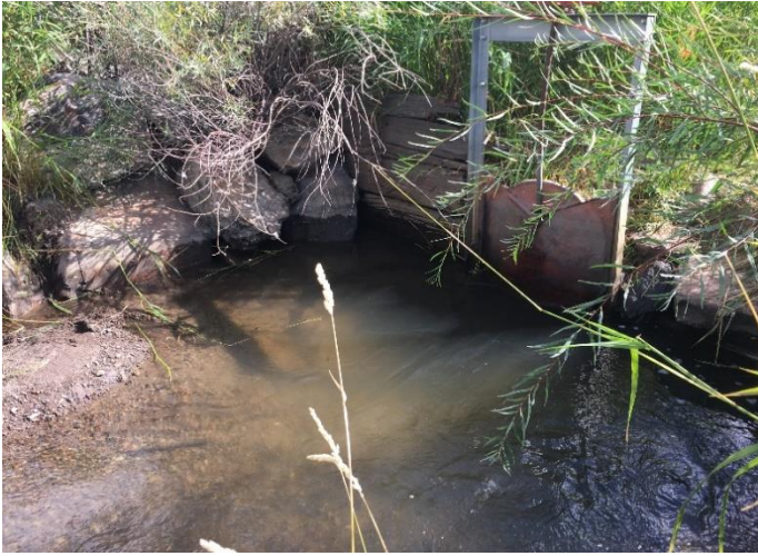
Headgate looking downstream
