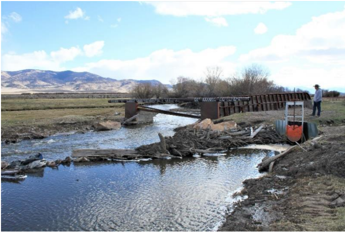
Headgate looking downstream
